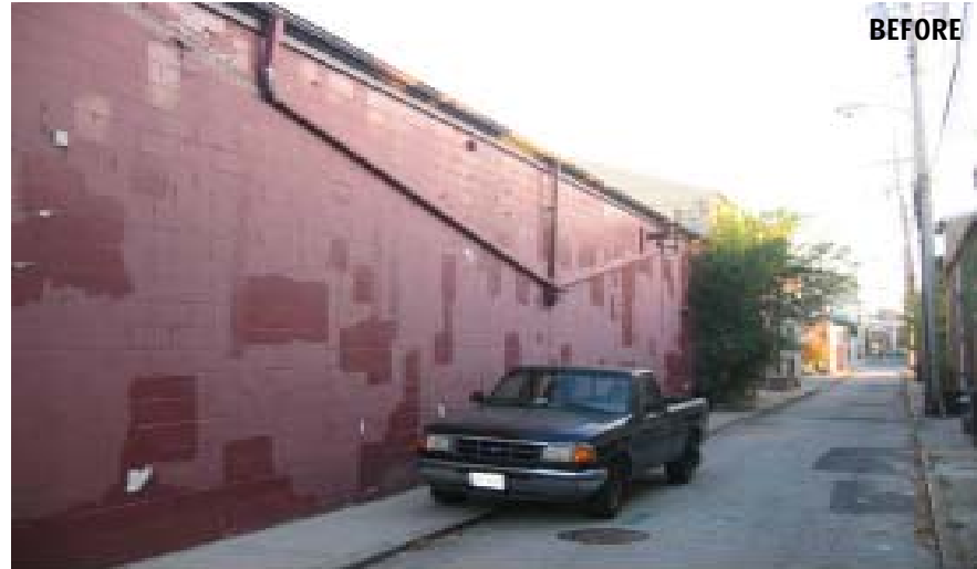
Side of existing warehouse, view looking southeast on Dallas St. from Bank St., to be replaced by new building facade below.
